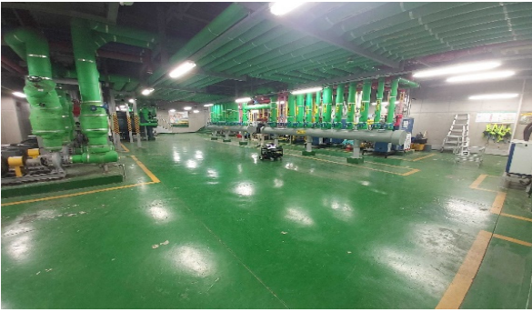
[Fig. 14] Experiment 3: Indoor facility environment 2
