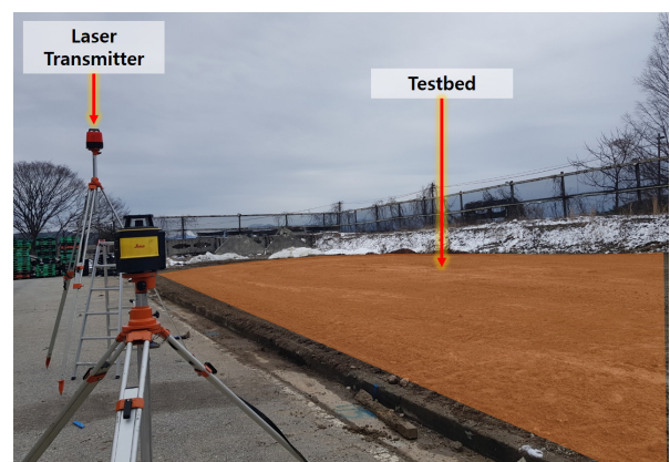
[Fig. 2] Installation location of the laser transmitter
